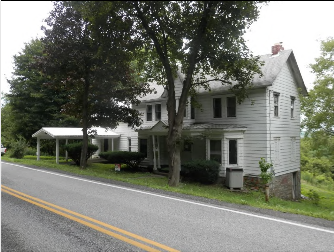
PHOTO 1: Exterior of the structure generally looking northeast
