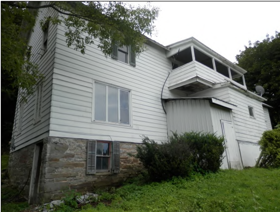
PHOTO 2: Exterior of the structure generally looking northwest
